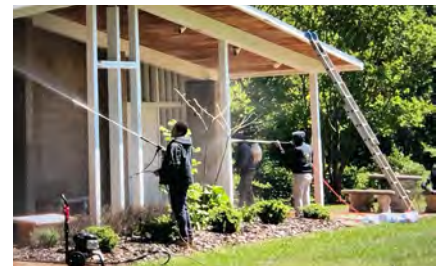
Members preparing Carolina Pines buildings for painting
